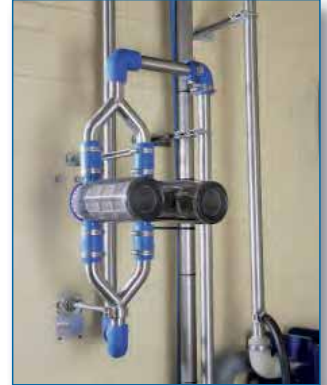
Twin FlowFilter Installation
